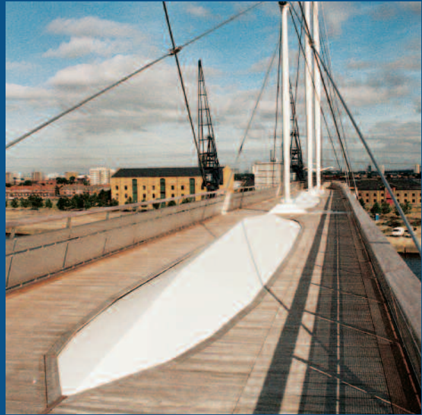
Royal Victoria Dock footbridge
